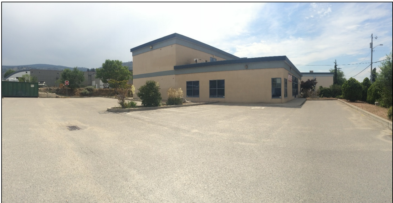
Figure 5 – Looking at north end of existing building at 2250 Camrose Street (within parking lot)
