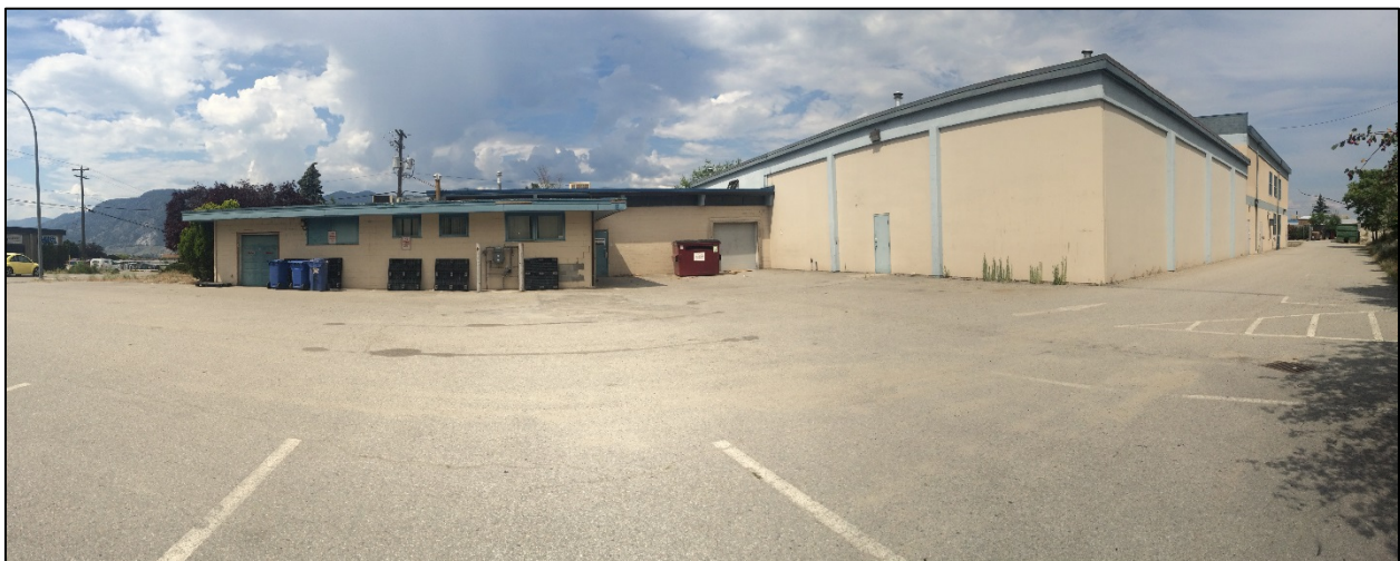
Figure 7 – Looking at the east wall of the existing building at 2250 Camrose Street
